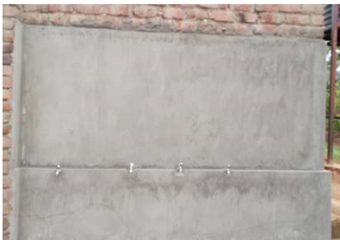
Another fill station
