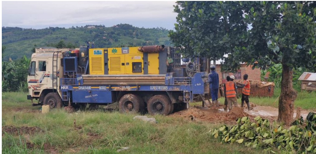
Well drilling truck and workmen
